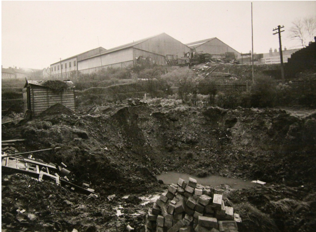
A black and white photograph showing bomb damage following an air raid at Tantany Estate, West Bromwich 10th November 1940. Photographer: Sidney Darby; from Sandwell Archives.
